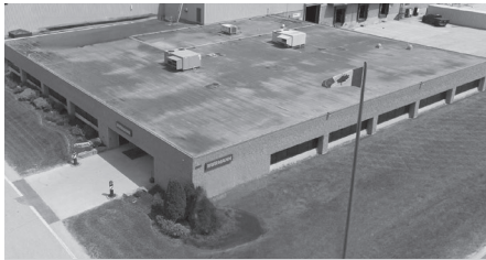
Barrie, ON (CAN) - High Performance Doors
