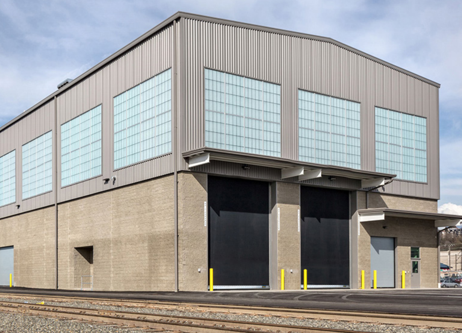
MODEL HD-DD 3065 in a rail transit maintenance facility
