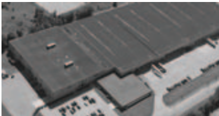
Barrie, ON (CAN) - High Performance Doors
