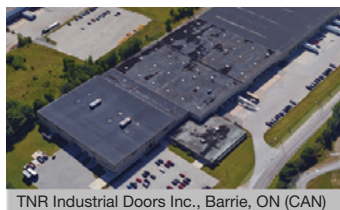
TNR Industrial Doors Inc., Barrie, ON (CAN)
